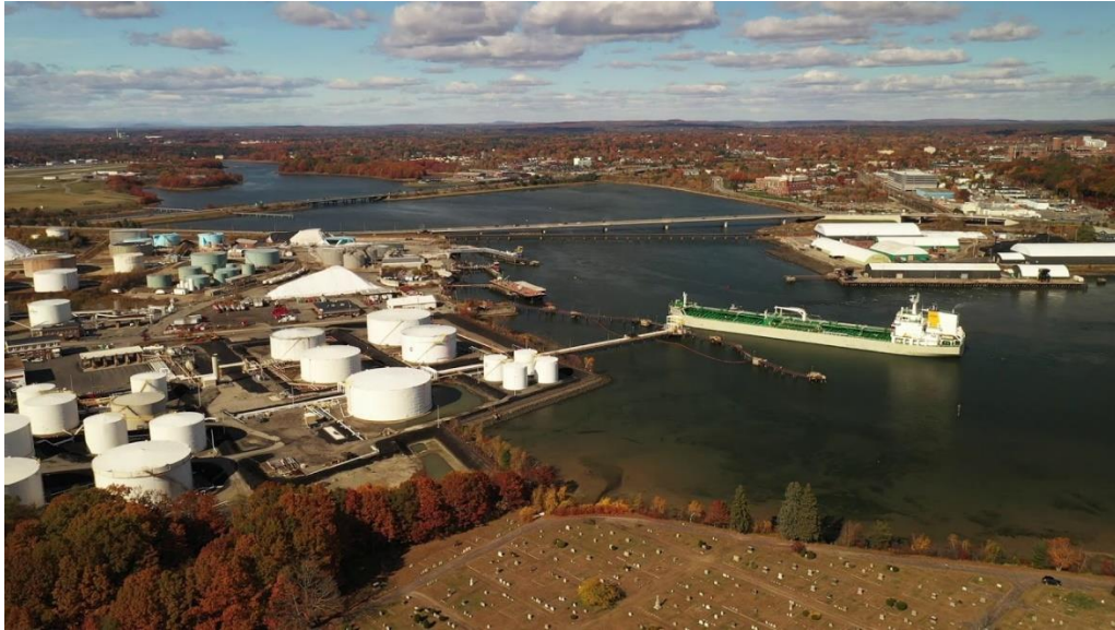
Figure 1 Aerial image of Forest City Cemetery and Sprague terminal in South Portland. Image courtesy of Inside Climate News.
