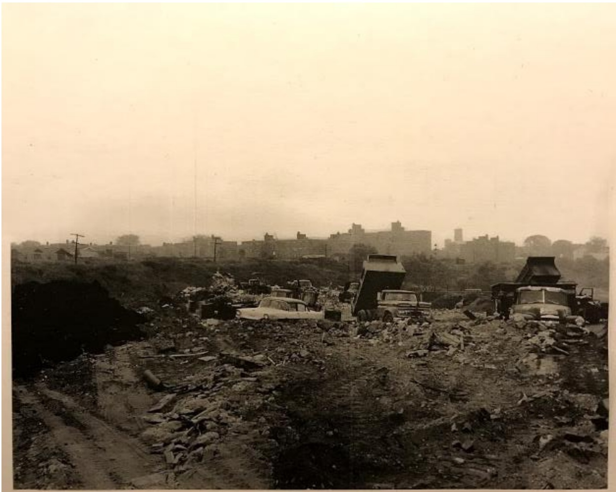
Figure 5 1962 photo of municipal dump trucks unloading in the Cambridge City Dump. Image courtesy of Cambridge Historical Commission.
